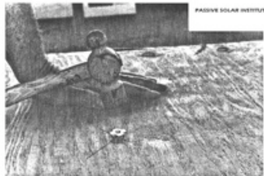
Insert T-nut and set with hammer
