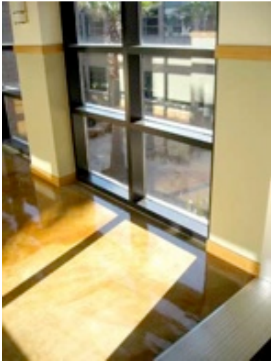
Exposed stained and polished concrete floor
