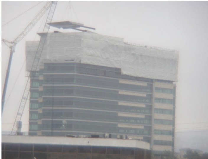
Top two stories being removed
