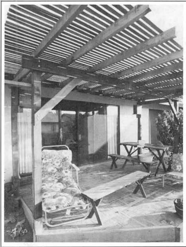
Photo V-3: A simple and nice looking patio overhang greatly reduces the solar gain to the west wall of this house, and it keeps the patio a little cooler too. The slats could also be crisscrossed to increase the shading effect.
