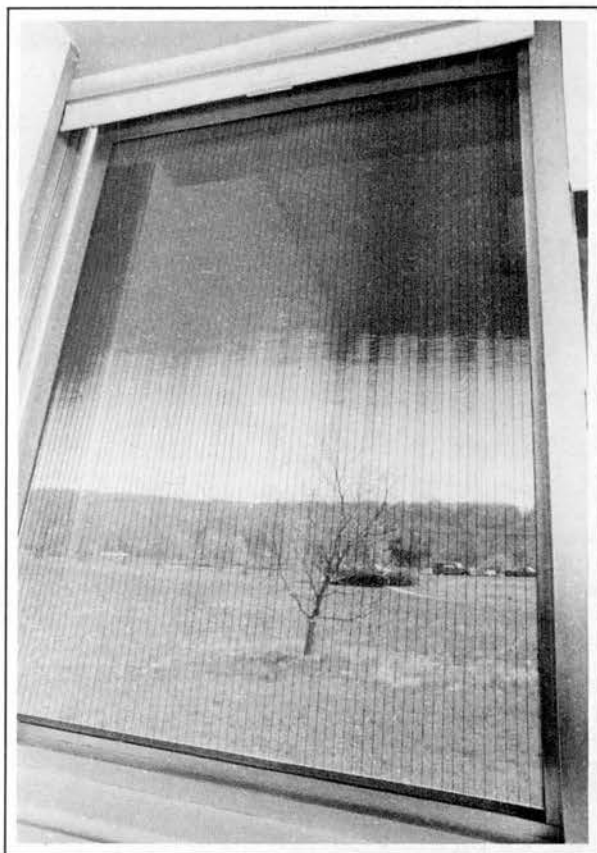
Photo V-5: Shade screens block sunlight, but they don't block the view. The photograph on the left shows the view through the screen at eye-level, while the one on the right shows how light is blocked when it comes in from a high (summer sun) angle.
