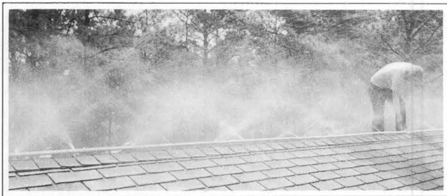
Photo V-7: Talk about unusual, a roof spray system in action is certainly a unique sight, but it may well become standard equipment for roofs in the not too distant future.
