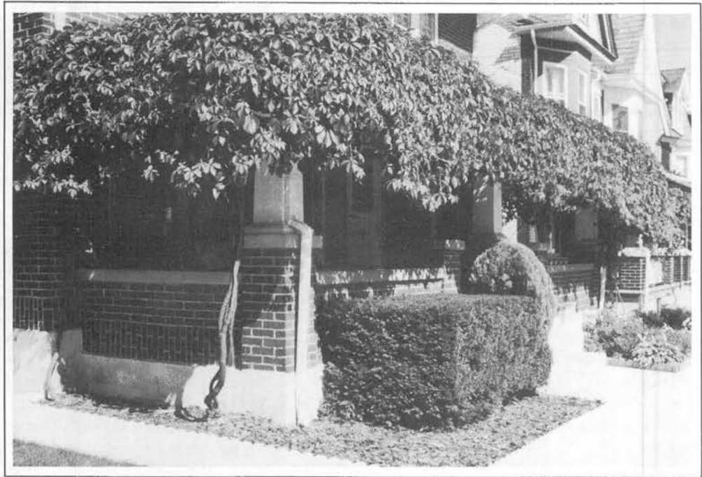
Photo V-6: These arbors are retrofits, of a few decades ago. The structure is formed of bent and straight pipe sections that are covered with a mesh that carries the grapevines.
